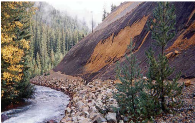
Regrade tailings and waste rock piles to prevent leaching into Railroad Creek
