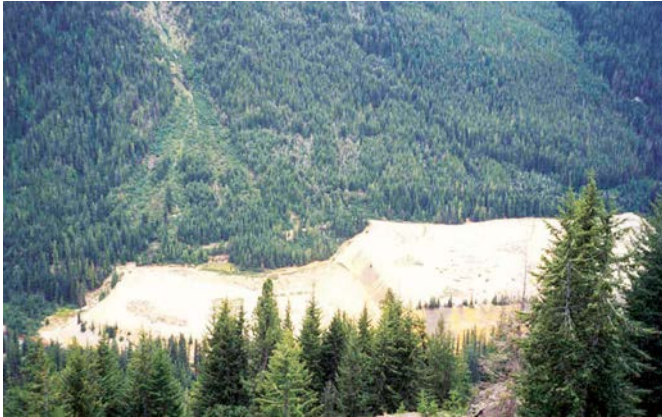
Cap re-graded tailings with crushed stone and growing medium, then plant
