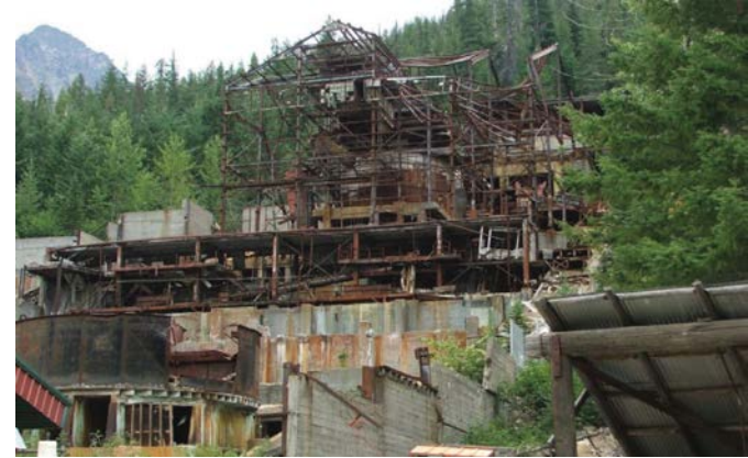
Demolish mill building
