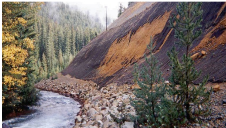
Regrade tailings to prevent leaching into Railroad Creek
