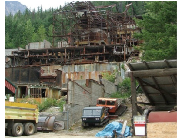
Demolish mill building
