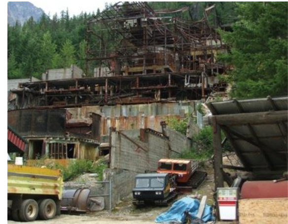
Demolish mill building
