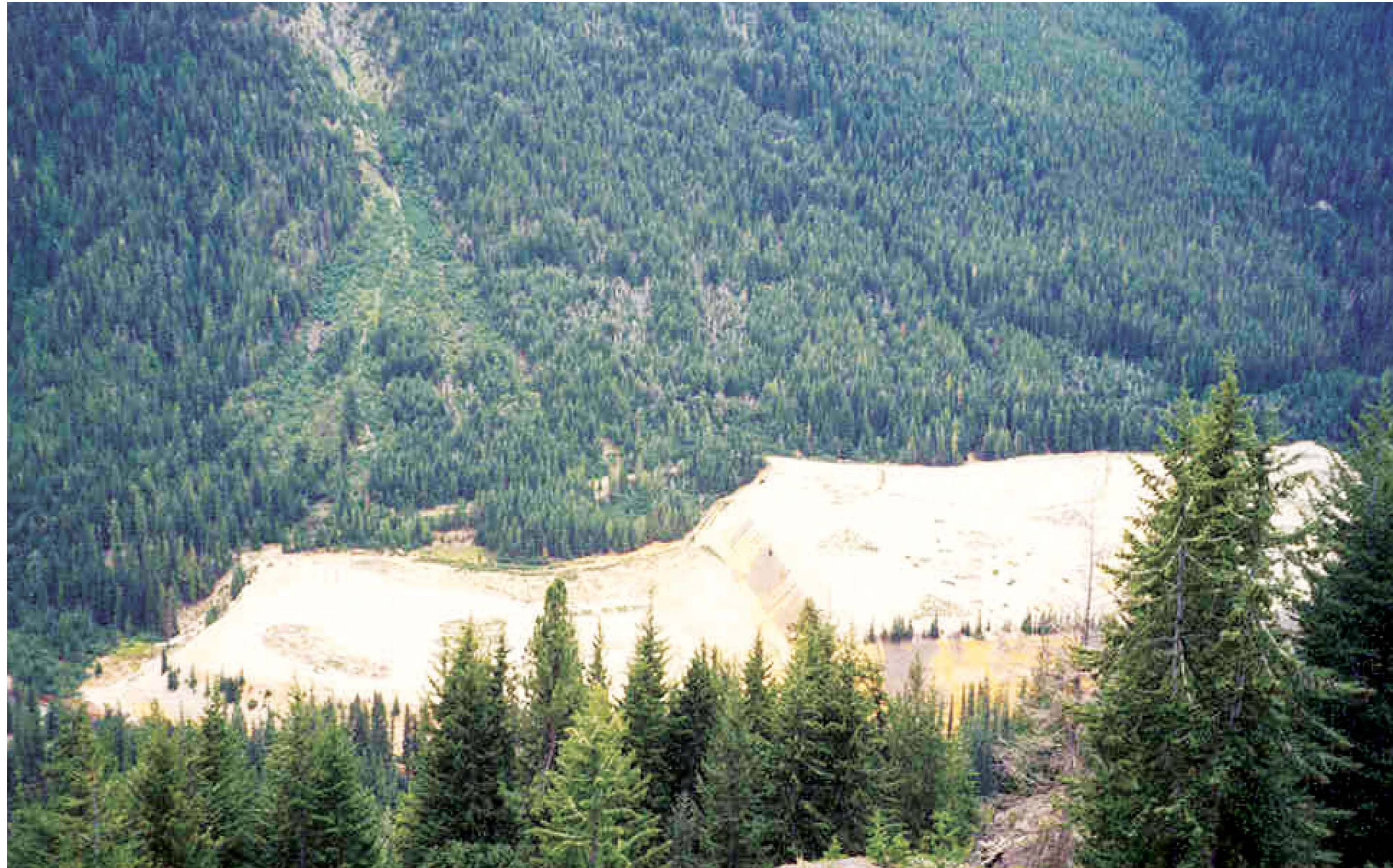
Regraded tailings will be capped with crushed stone and growing medium, then planted
