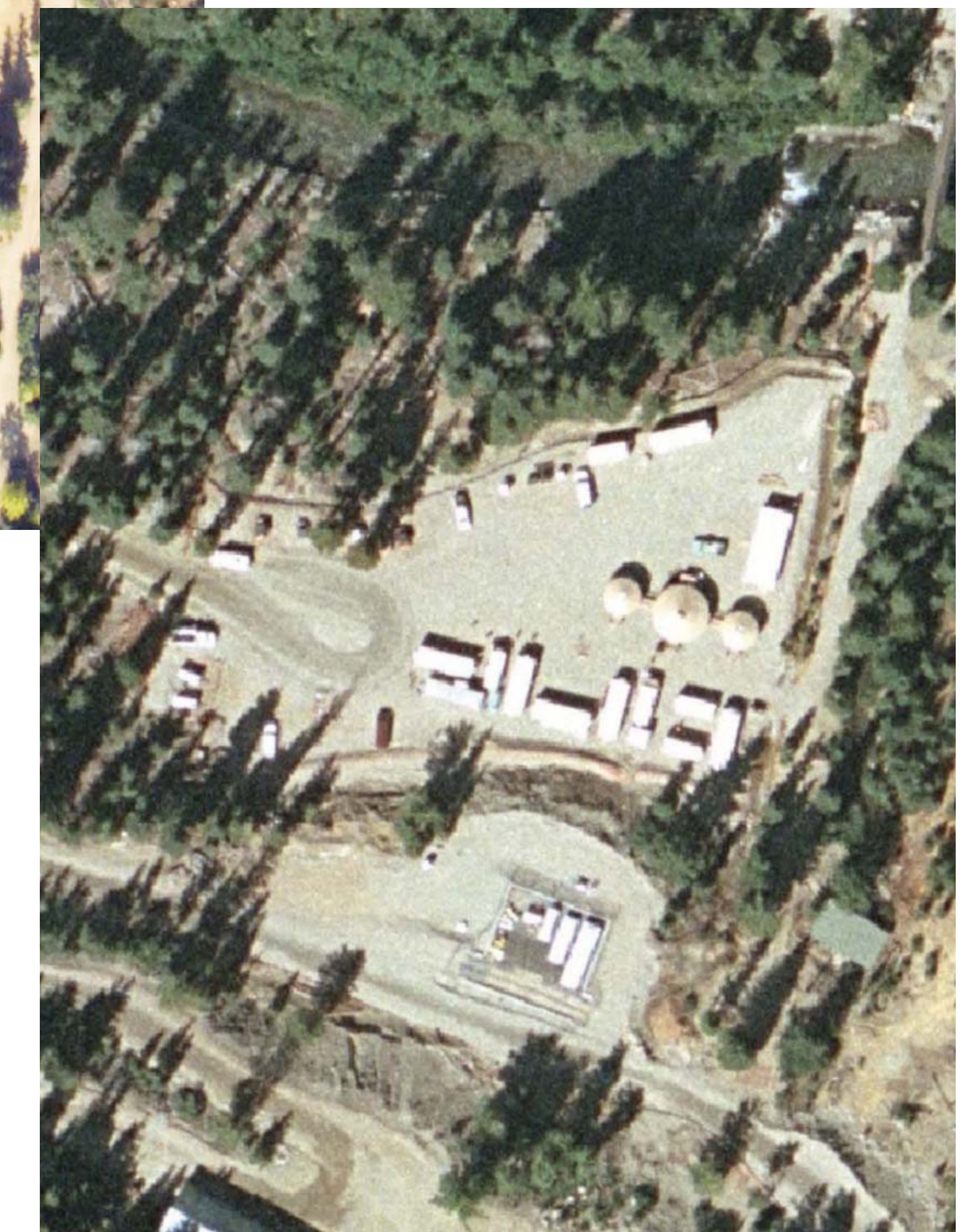
Contractor Staging Area
