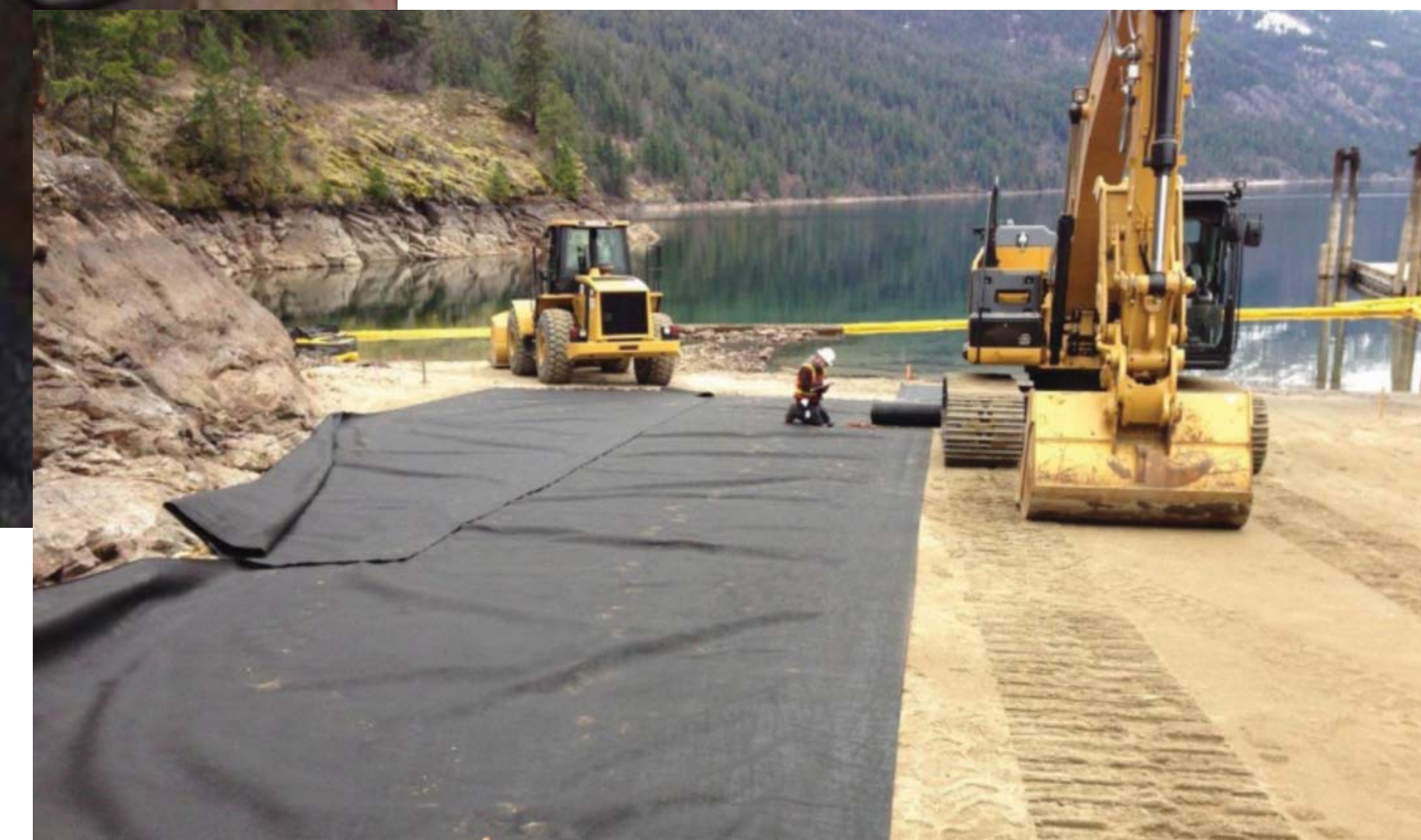
Barge Ramp Construction at Lucerne
