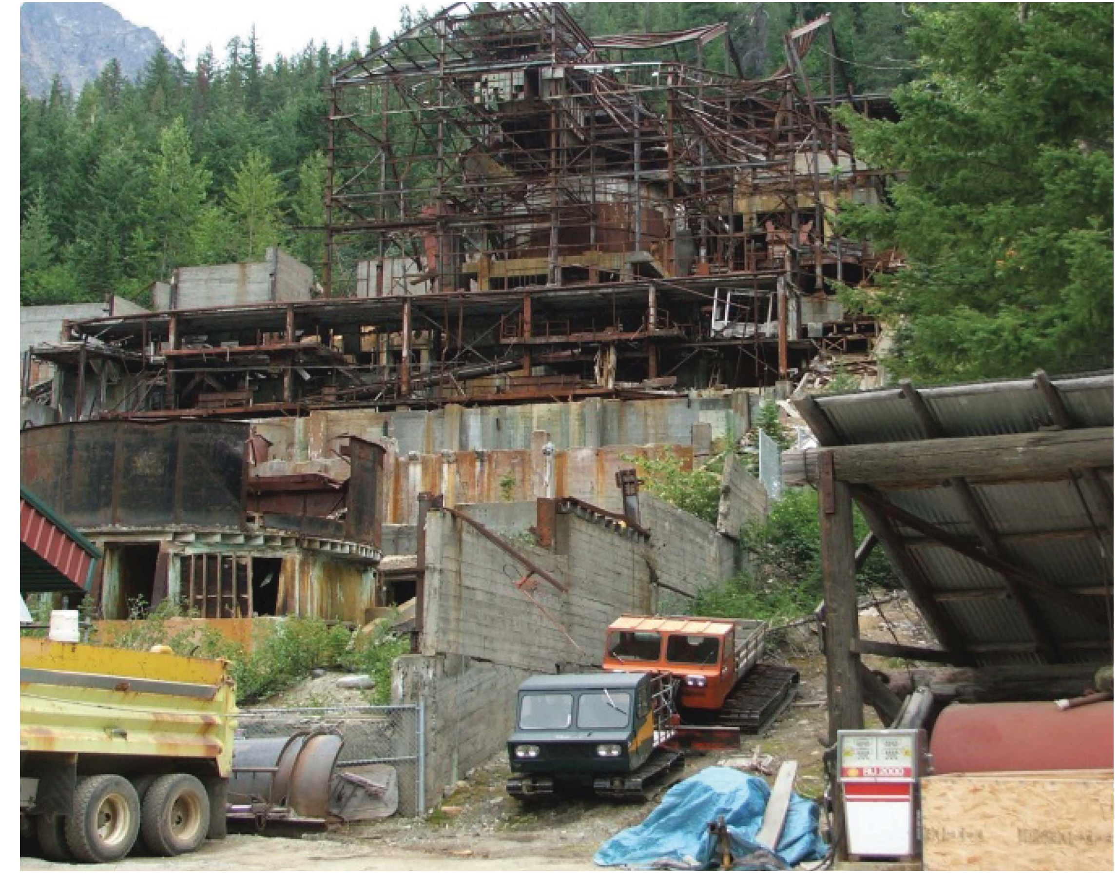
Mill building will be demolished
